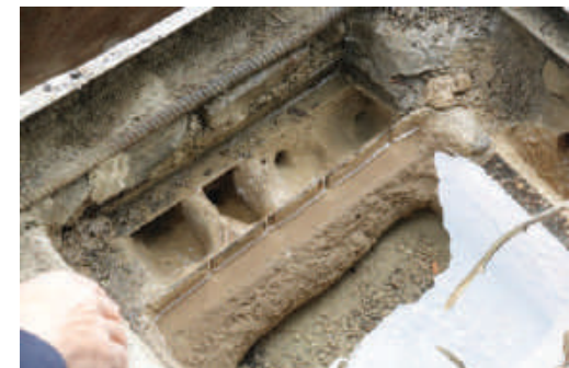
Figure 6. Distribution well with comb distributor
